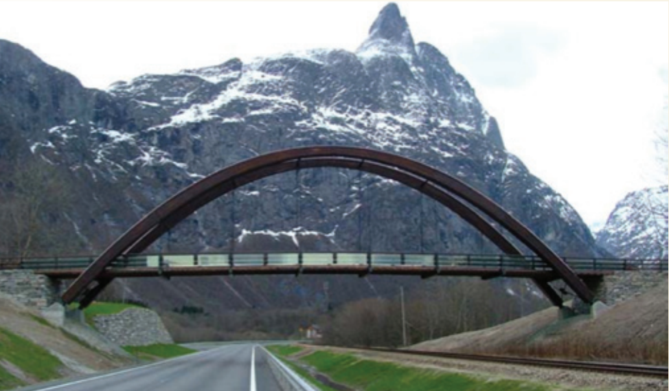
Ner-Hole (Romsdalsporten) Bridge Span: 42 m. Construction year: 2006.
