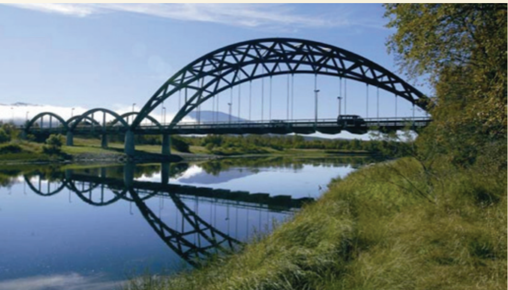
Tynset Bridge Main span: 70 m. Construction year: 2001.
